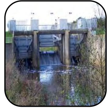
Figure 13 Leigh barrier gates
