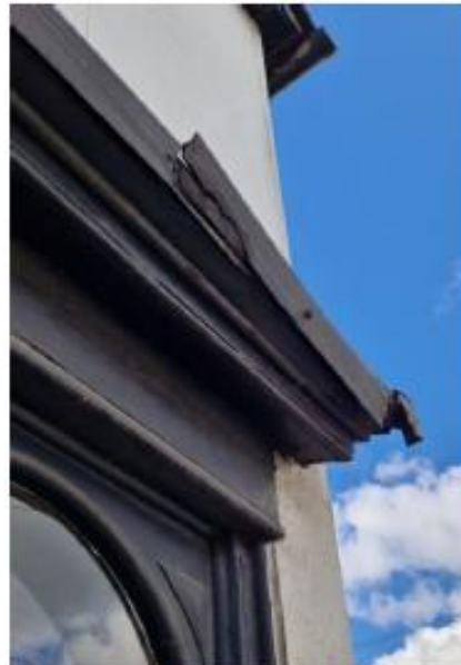
Figure 12. Damage to historic building in the conservation area as a result of passing large vehicles on the very narrow street.
