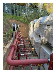
**Larkfield Leisure Centre:** air source heat pumps (ASHP) being installed as part of the decarbonisation programme, partly funded by the Public Sector Decarbonisation Scheme (PSDS). Completion expected by April 2026.
